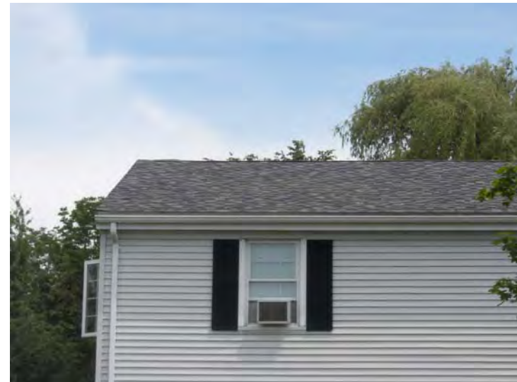
Asphalt shingle roofing in good condition
