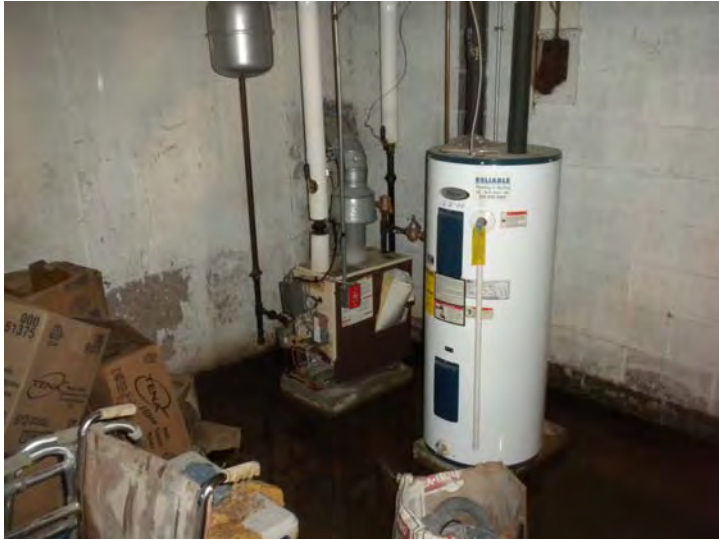
Typical boiler and domestic hot water configuration
