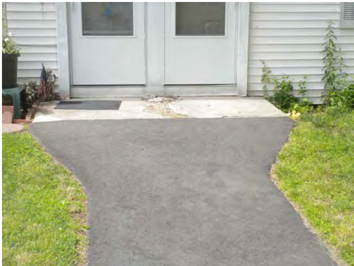
Example of spalling concrete at the unit entrance pad
